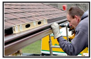
Leafaway gutters are installed without driving nails or screws into your roof and without lifting your shingles so not to void your roof warranty. Our gutter protection system is screwed to the fascia board with internal hanging brackets, unlike conventional gutters that are attached with spikes and can come loose.
